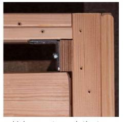
Make sure to push the top slat as far up as it can go, and the bottom slat as far down as it can go. Both top and bottom slats have to touch the exterior frame. Screw in all the slats using the 40mm screws provided.
