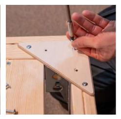
Screw it in place with the pozey flange screws provided.
